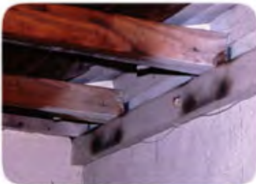
Rats activity clearly indicated by grease marks around rafters ( below ) and holes in walls ( above )
